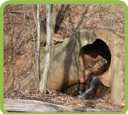
An existing stormwater outfall from Interstate 64 near the Old Mills Trail. This type of facility is discouraged.
